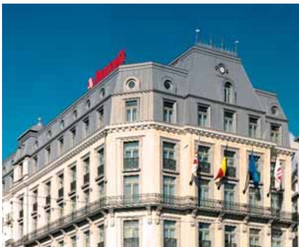
Arch. B. Delwarde – QUARTZ-ZINC®
